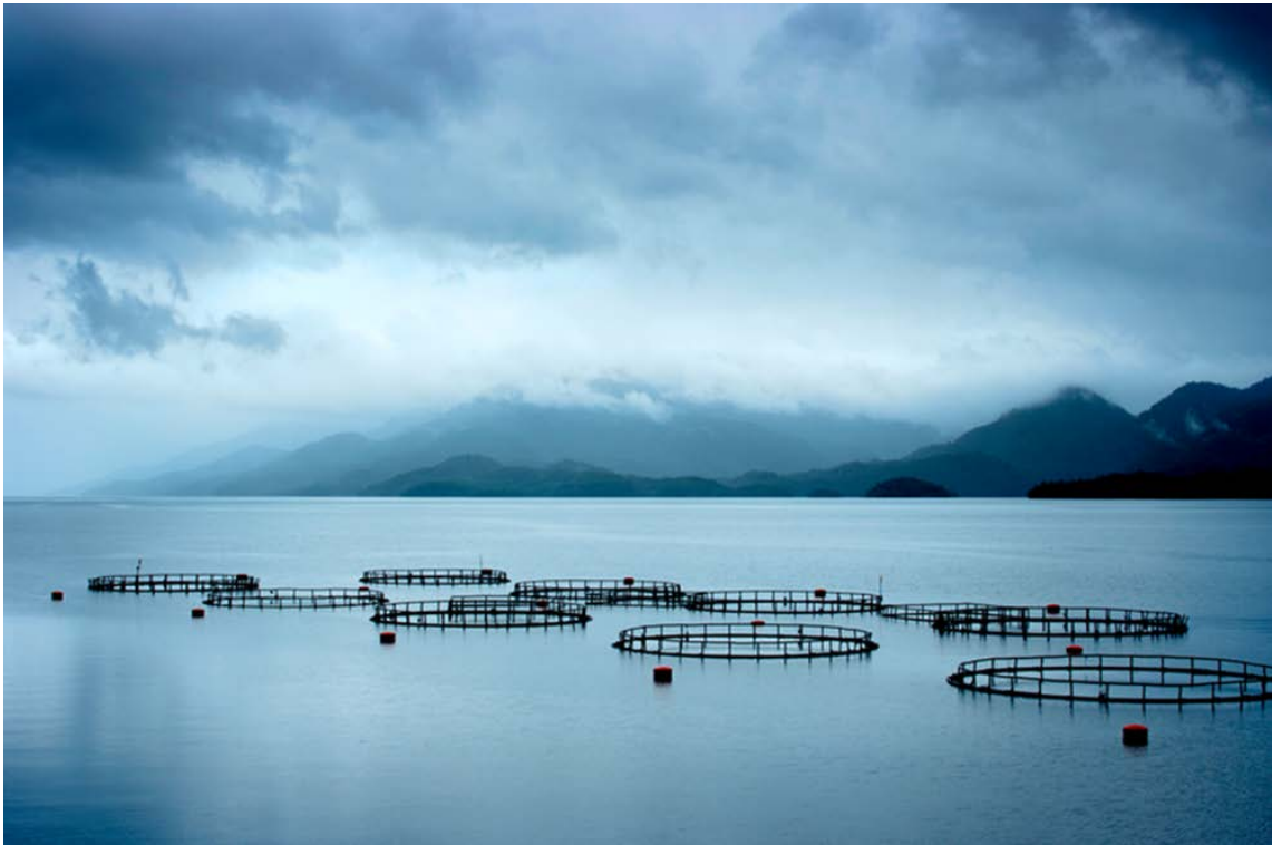
Figure 20 About 50 % of fish farms in Norway get power from shore. It is commercially profitable to electrify 80 % of the Norwegian production.
